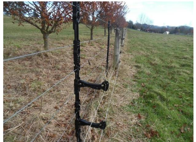
We purchased the 7 strand styx (they come in a range of sizes) and also the outriggers. We easily applied these to the fence. Each styx has several options of twisting and securing the outrigger and no special equipment was required other than elbow grease!
